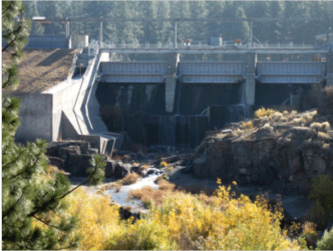
H&N file photo by Jill Aho J.C. Boyle Dam is one of four dams on the Klamath River that would be removed as part of the implementation of the Klamath Basin Restoration Agreement.
